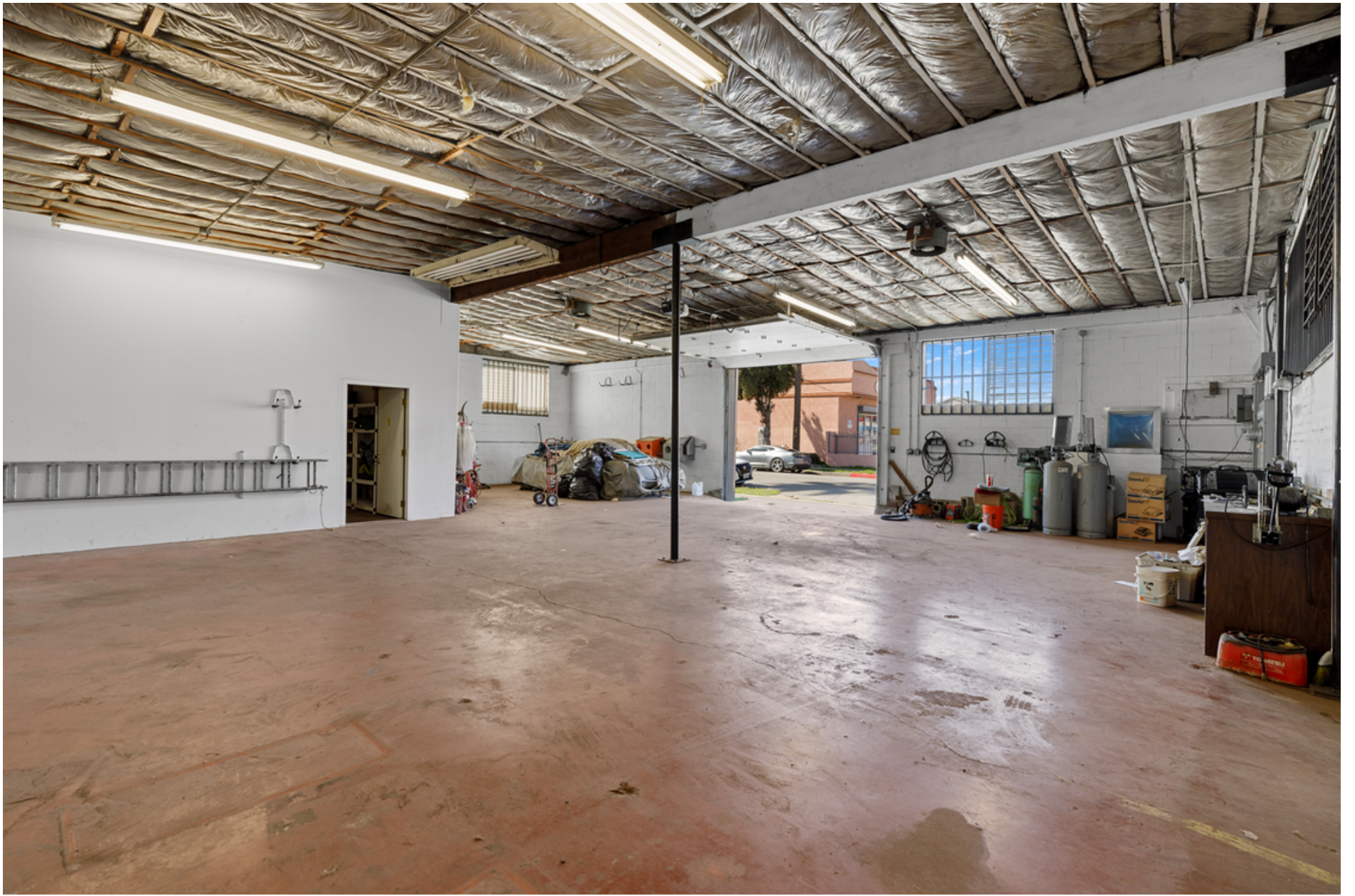
Warehouse - Open Layout and Ceiling Height
