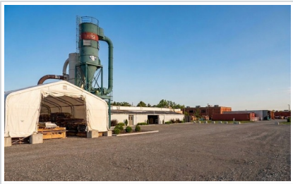
Rear yard and dust collection system
