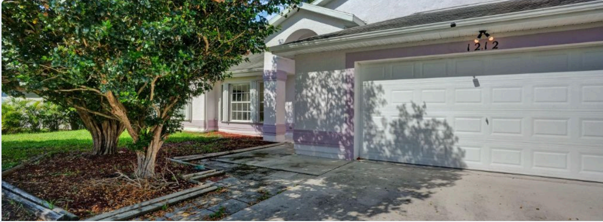
EXTERIOR / FRONT FACADE
