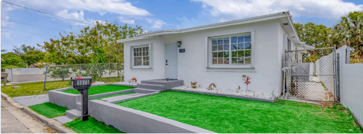
EXTERIOR / FRONT FACADE
