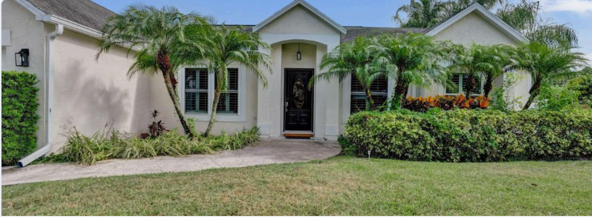
EXTERIOR / FRONT FACADE
