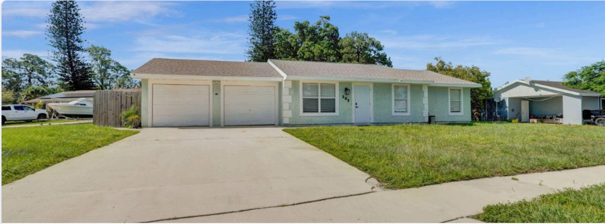
EXTERIOR / FRONT FACADE
