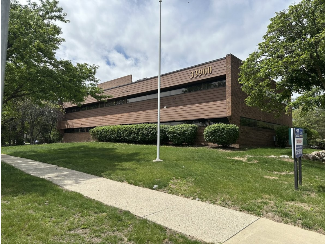
EXTERIOR · SCHOOLCRAFT ROAD FRONTAGE
