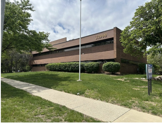
CURRENT CONDITION · SCHOOLCRAFT FRONTAGE
