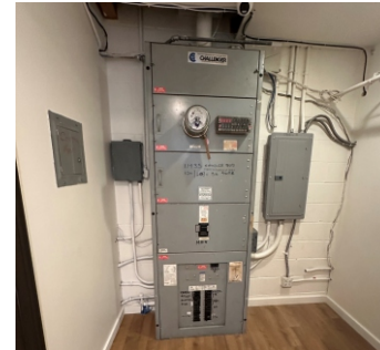
Main Panel is 400 amps and there are Two Sub Panels which are 200 amps each
