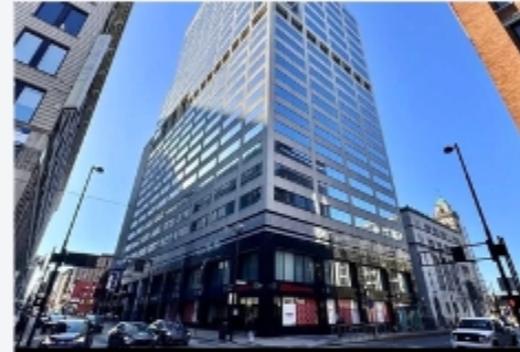
The Avant Office Conversion Project
