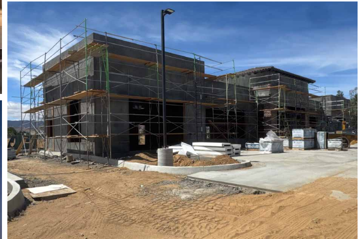
Construction — In Progress
