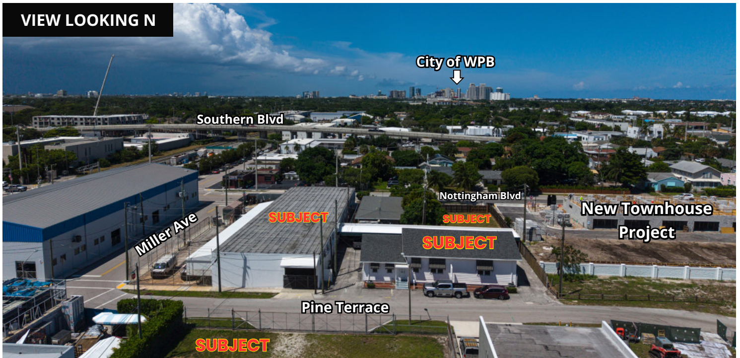
VIEW LOOKING N
