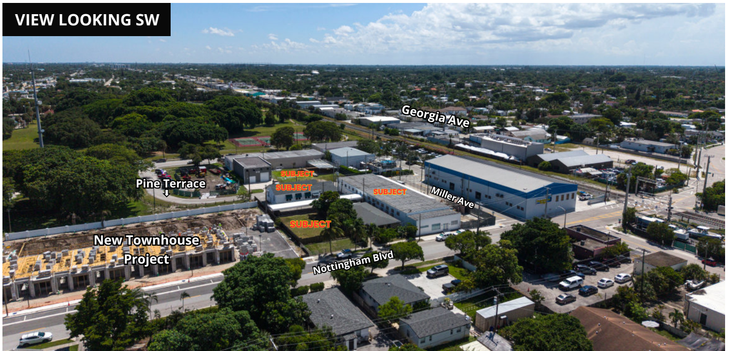
OVERHEAD VIEW LOOKING SW
