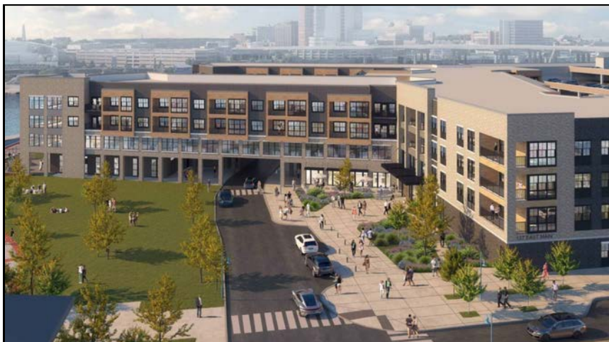
THE AUGUST AT STEELPOINTE HARBOR
