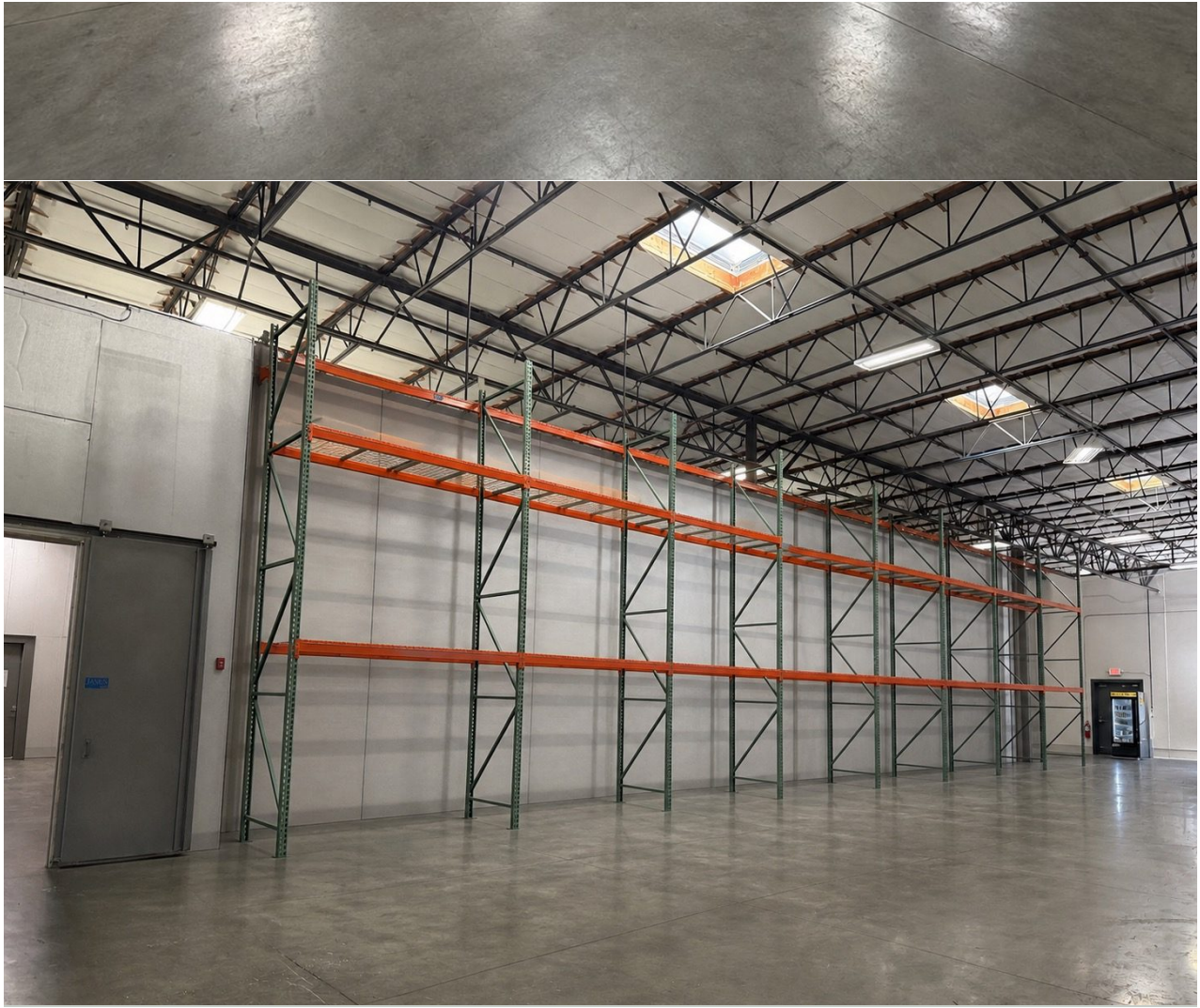
WAREHOUSE — PALLET RACKING IN PLACE, TILT-UP PANEL WALLS, WALK-IN COOLER AT LEFT
