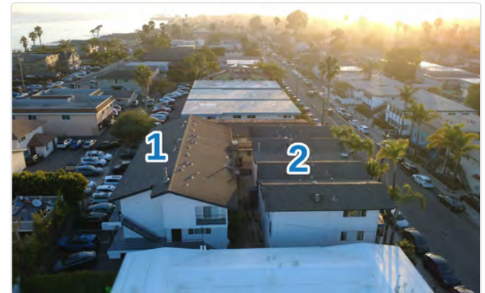
AERIAL VIEW · BUILDING 1 & BUILDING 2 19 UNITS ACROSS TWO STRUCTURES
