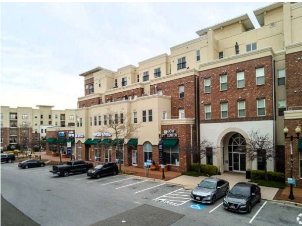
View of Shops at Midtown
