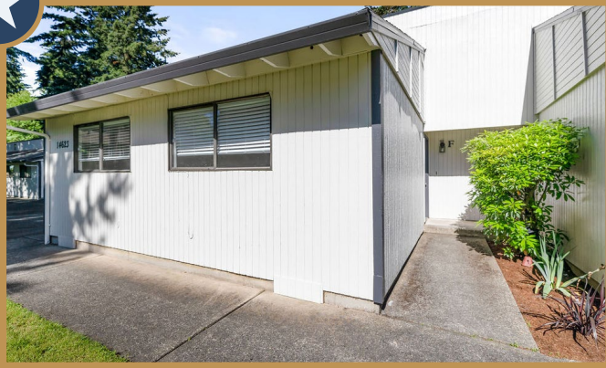
Coast Pine Apartments 14621-14625 NE Coast Pine Ct, Vancouver, WA
