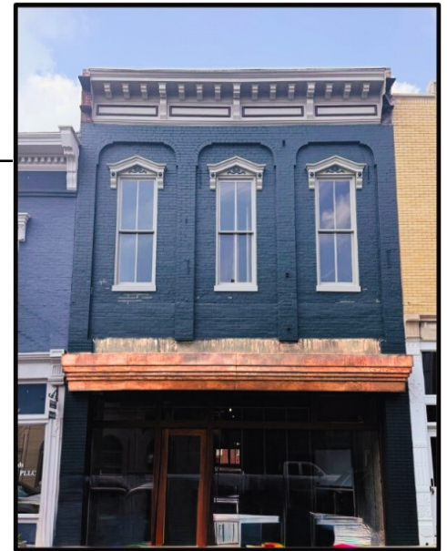
Exterior: Main Street Façade
