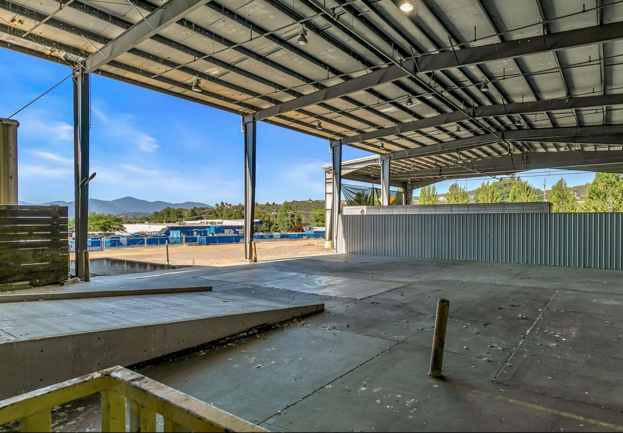
Awning NW Facing (Dock)
