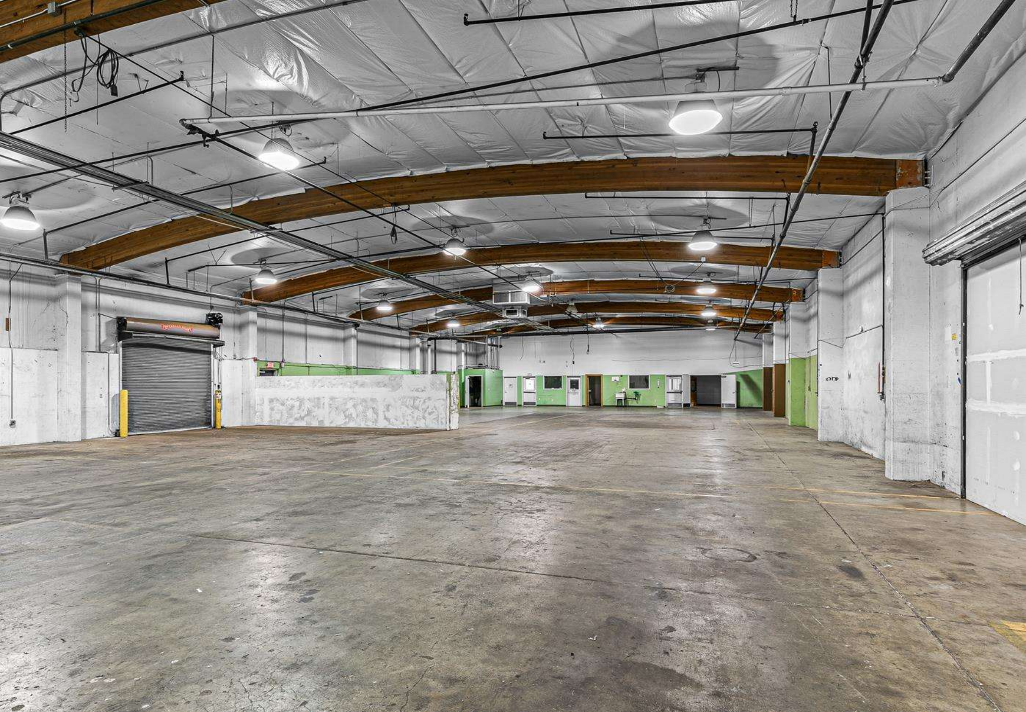
Interior Warehouse South Facing
