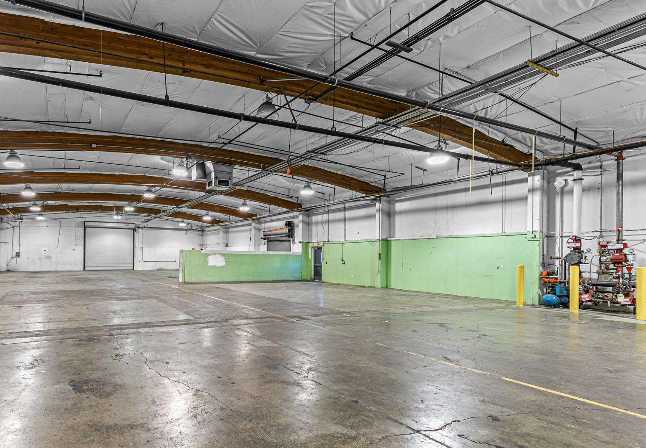
Interior Warehouse North Facing
