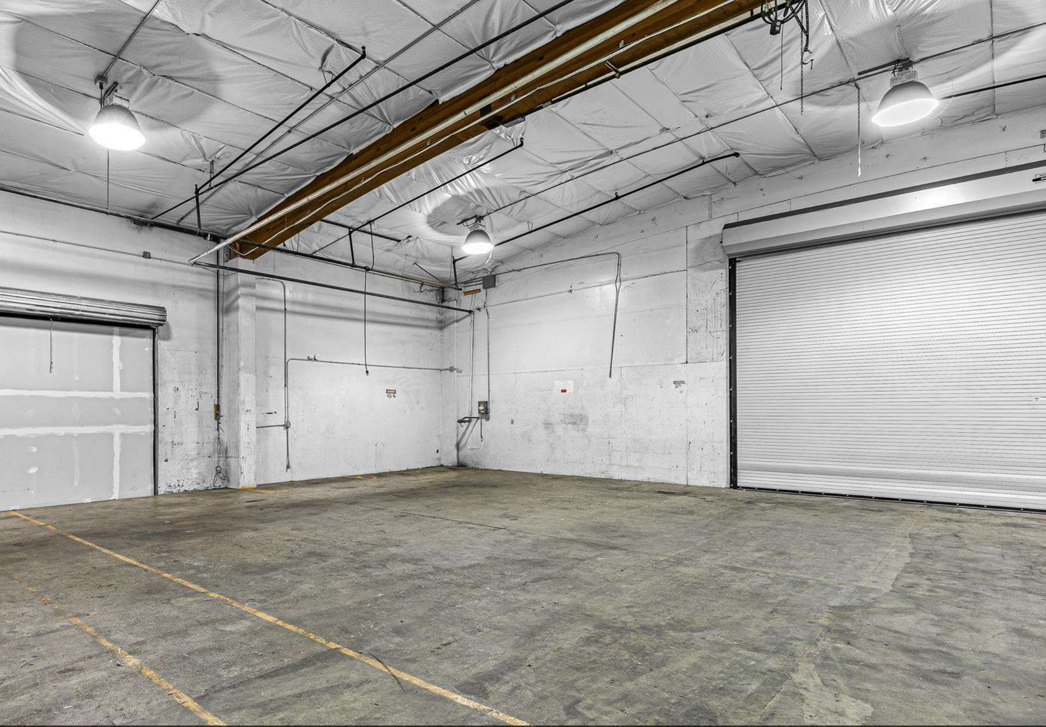
Warehouse NW Facing (1 of 3 Loading Doors)
