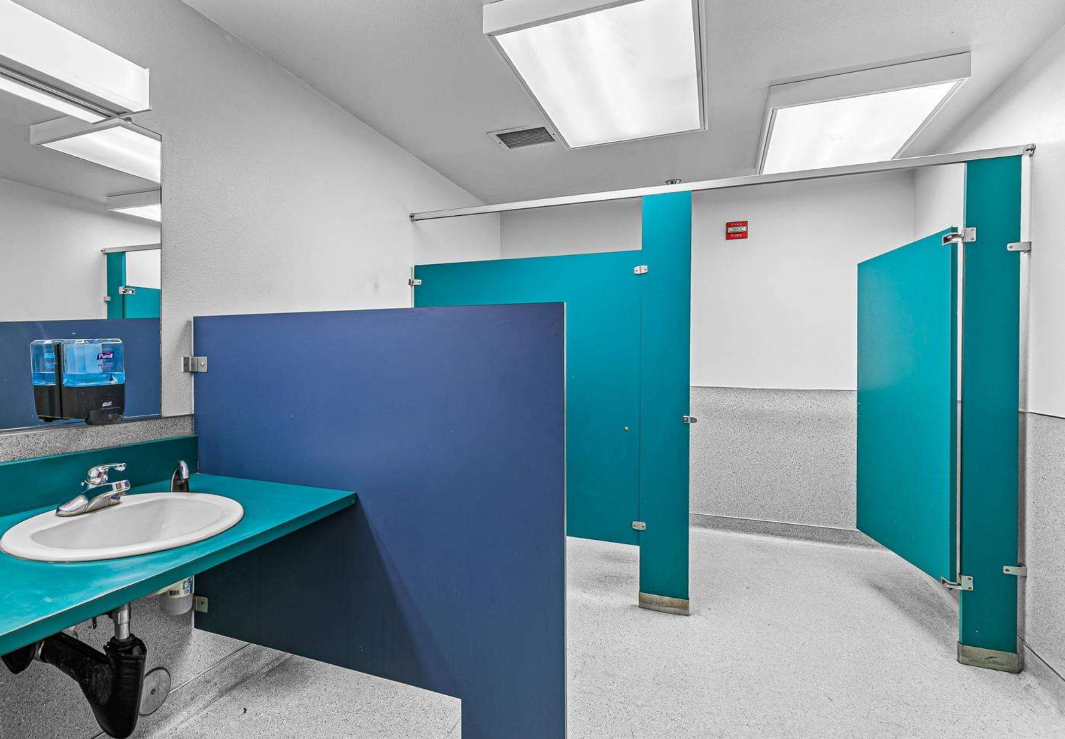
Men's Restroom (1 of 3 Restrooms)
