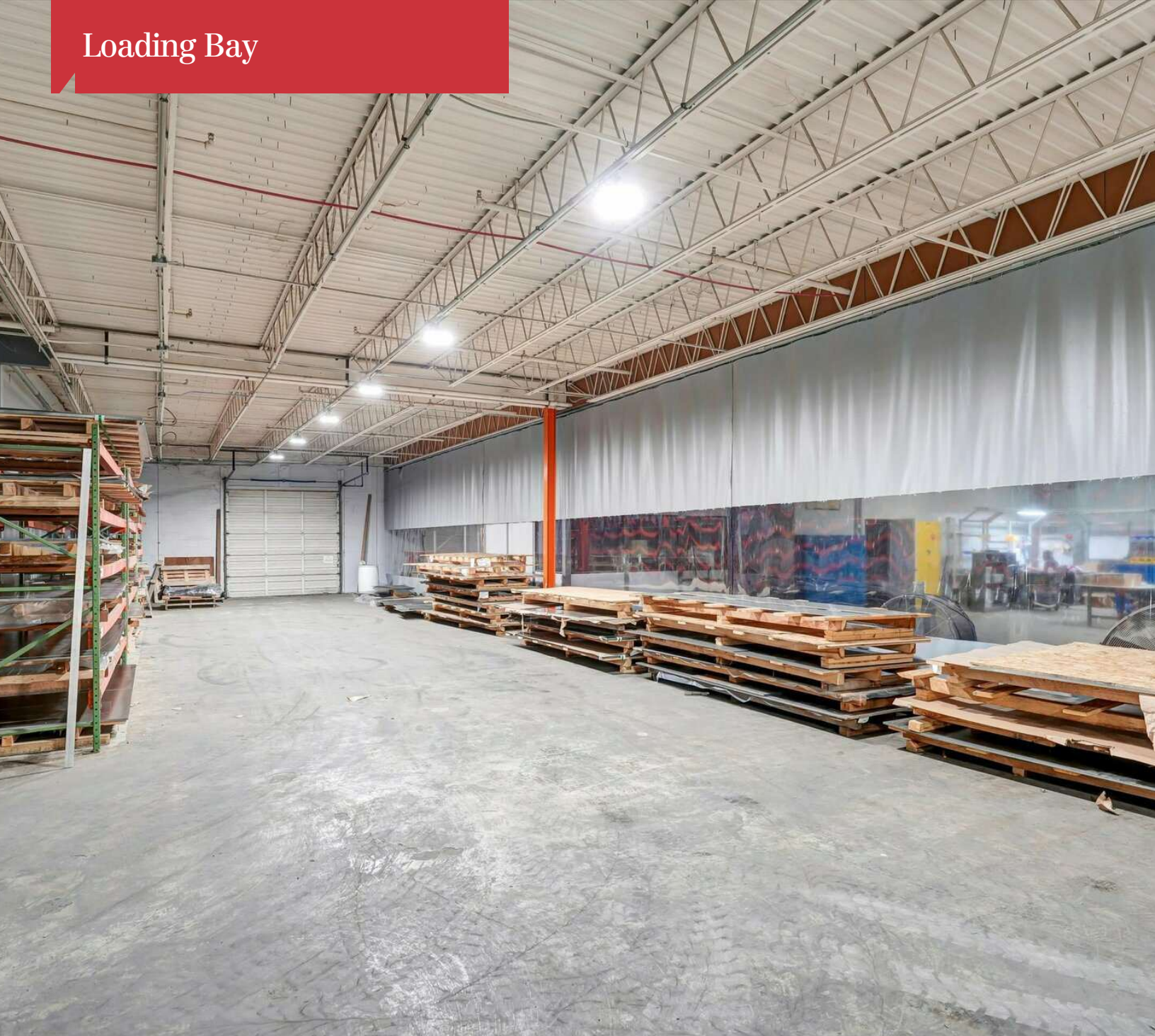
Dock high door that has been ramped for loading.
