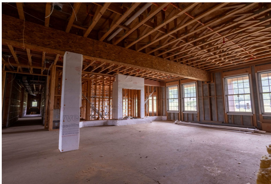
Interior framing and rough in. Windows installed, steel in place.
