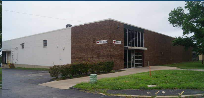
11688 Fairgrove Industrial Blvd Maryland Heights, MO 63043
