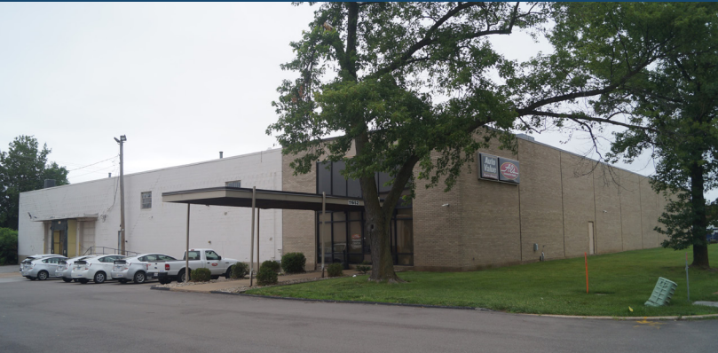
11652 Fairgrove Industrial Blvd Maryland Heights, MO 63043
