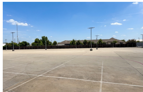
Secured rear lot — 40 car parks for storage, staging & employees
