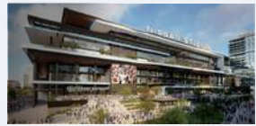
NISSAN STADIUM REDEVELOPMENT New $2.1 B Stadium 60,000 Seats
