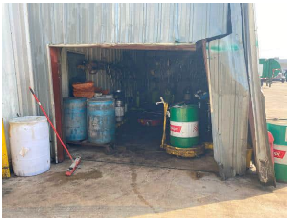
Photo 11 View of the on-site drum storage area (Tract 1)
