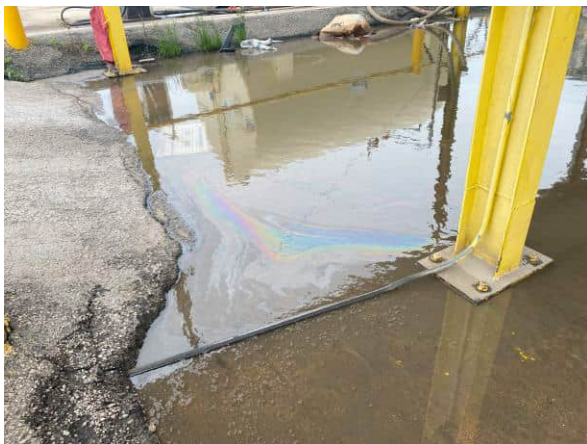
Photo 21 View of petroleum hydrocarbon sheen on standing water beneath the ASTs (Tract 2)
