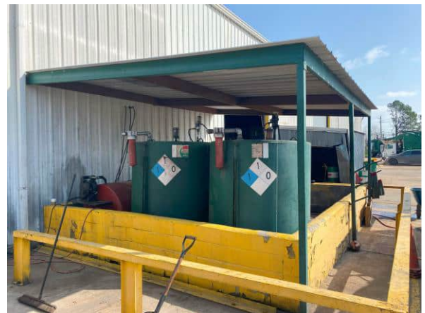
Photo 10 View of the on-site AST containment area (Tract 1)
