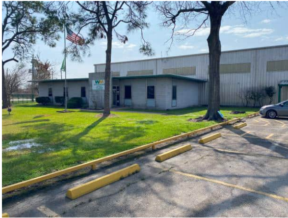
Photo 1 Typical view of the on-site office/warehouse building facing southeast (Tract 1)
