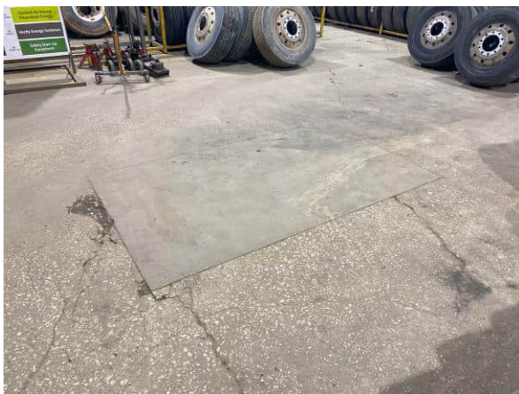
Photo 29 View of an apparent former in-ground hydraulic lift location (Tract 2)
