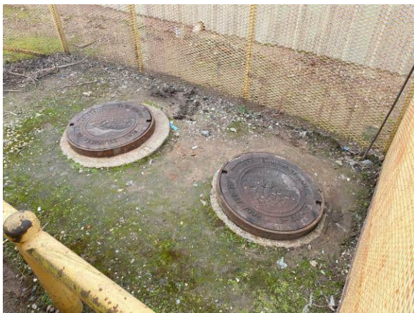
Photo 27 View of an on-site oil/water separator (Tract 2)
