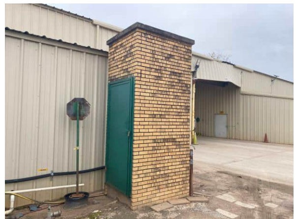
Photo 30 View of an on-site well house (Tract 2)
