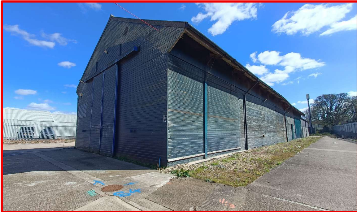
Timber framed building in the middle of the site
