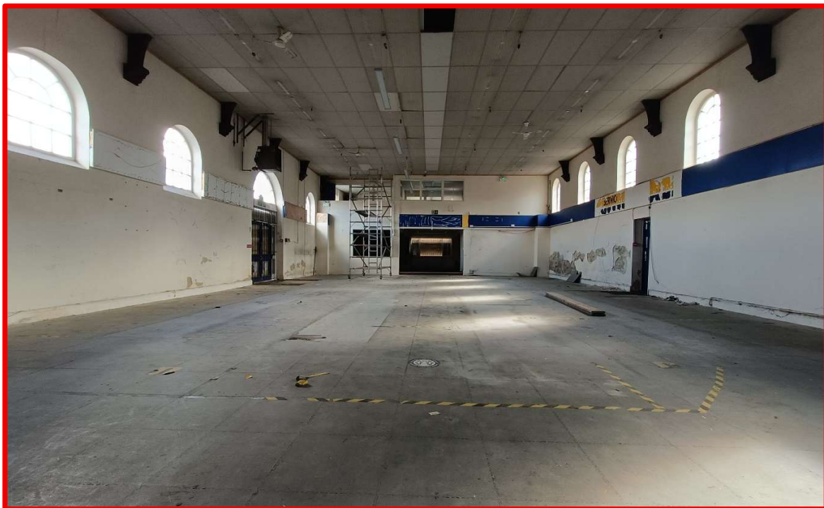
Internal photo of brick building
