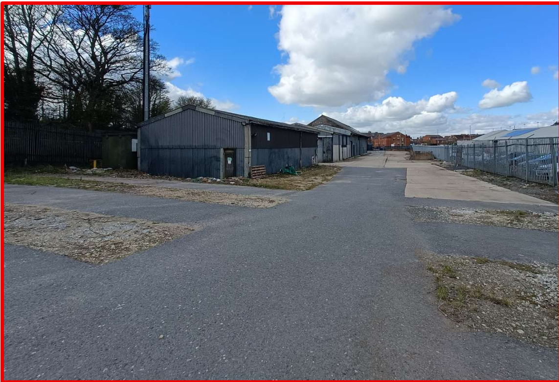
View of site looking towards main entrance
