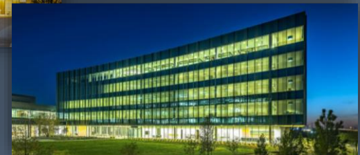
Anadarko Petroleum Building
