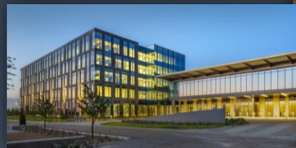
Occidental Petroleum Building
