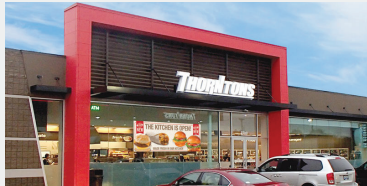
New Thorntons Gas Station
