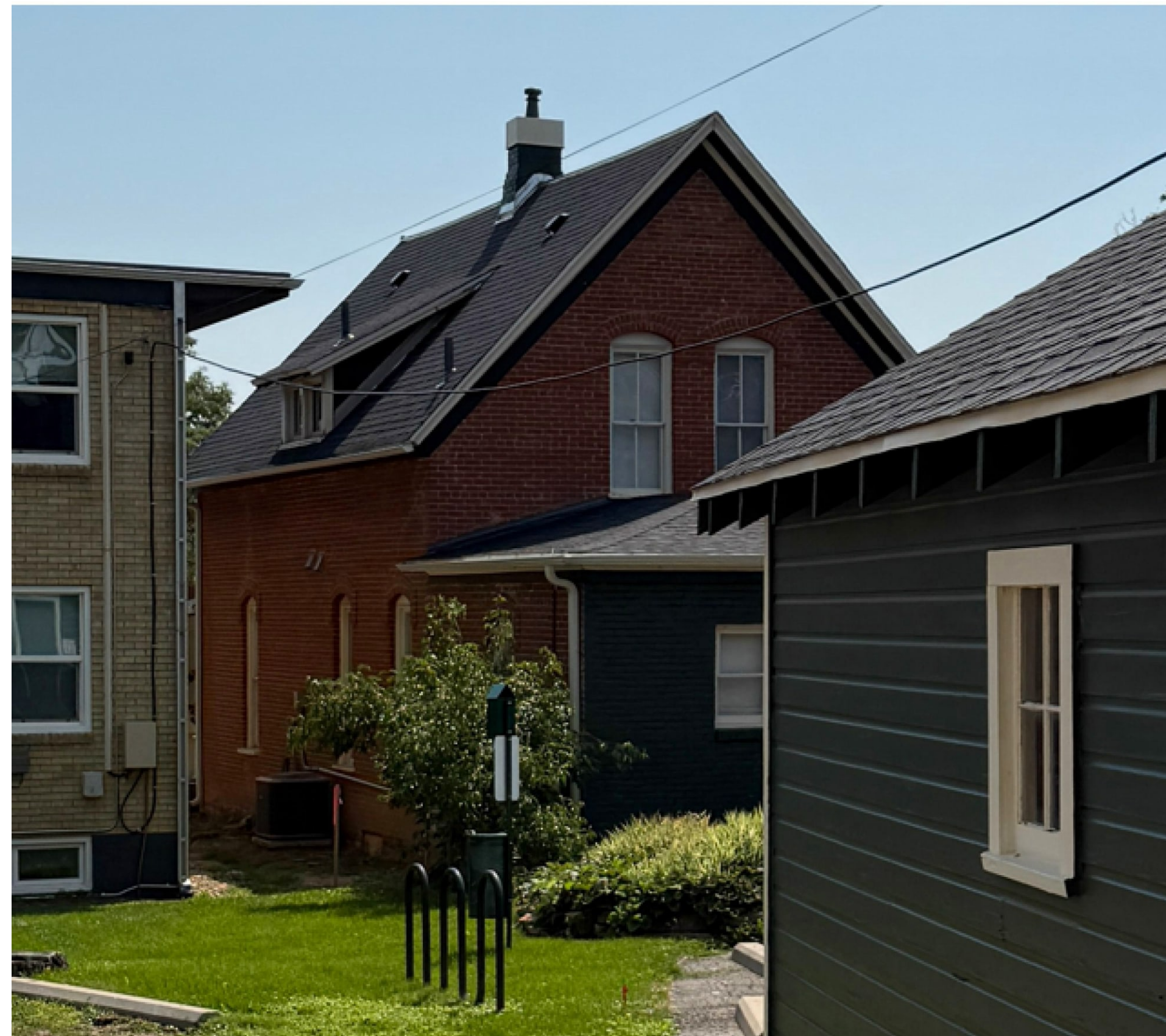
PHOTO FROM ALLEY (NORTHWEST)
