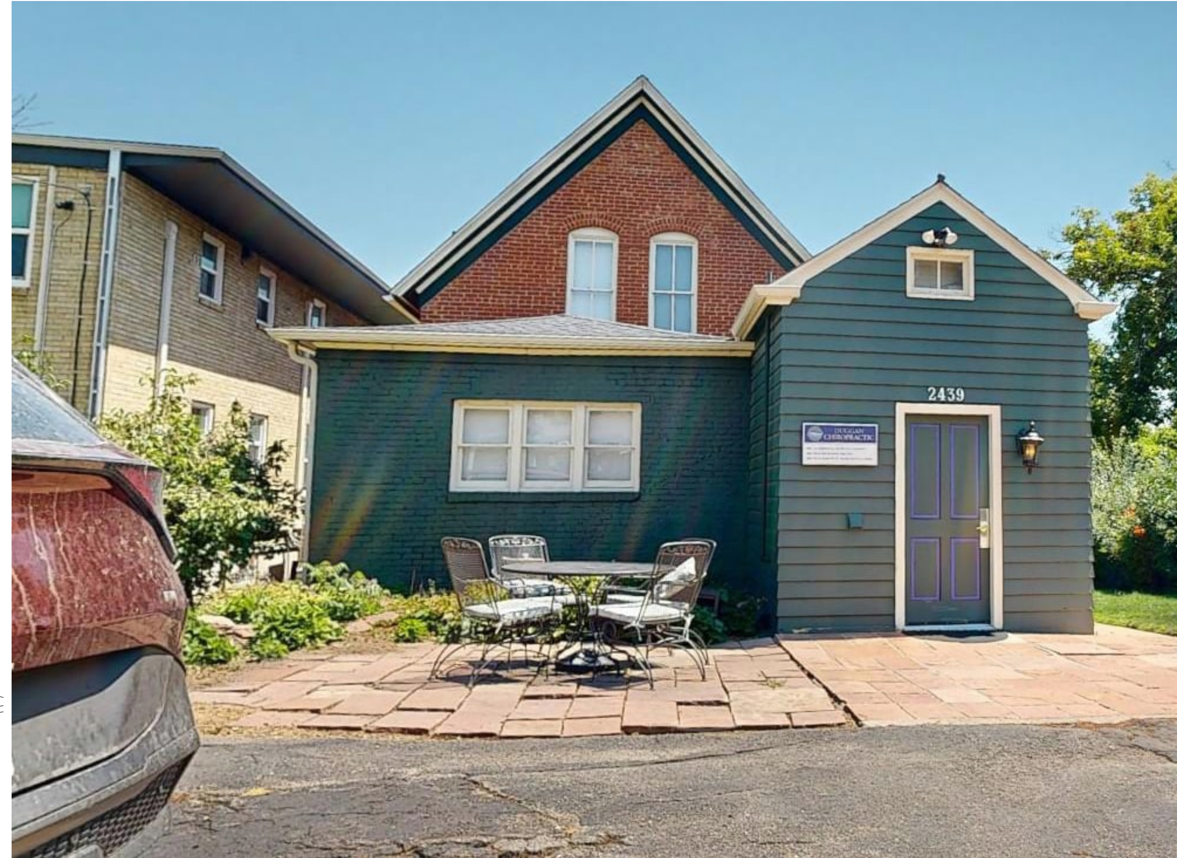
PHOTO FROM ALLEY (WEST)
