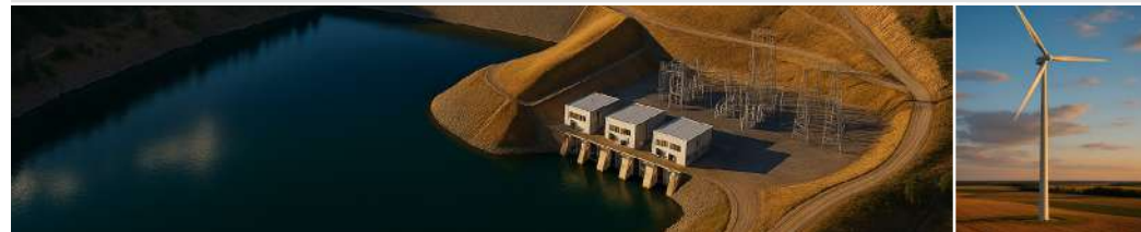
Cat Creek Energy and Water selects Voith Hydro for Idaho renewable energy and... Progress on Idaho's Cat Creek Energy and Water Project (Hydro Leader Magazine)
