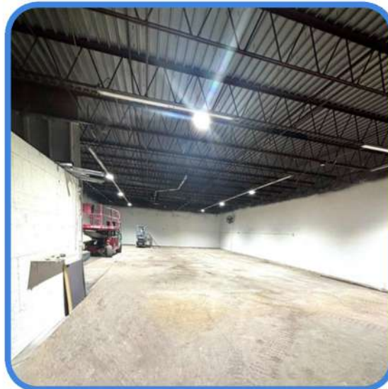
WAREHOUSE-1 WITH OFFICE
