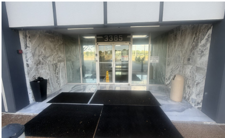
Lobby / Common Area
