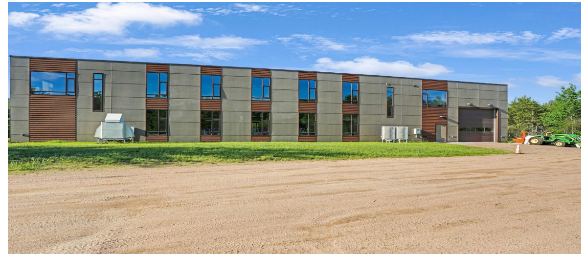
Rear elevation - grade-level bay door, ductless heat pumps and generator
