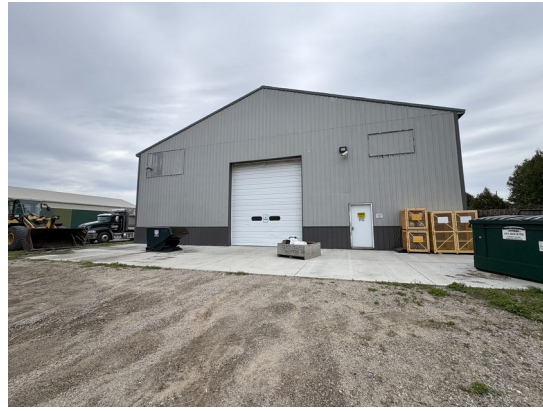
Exterior — West Bay Overhead Door
