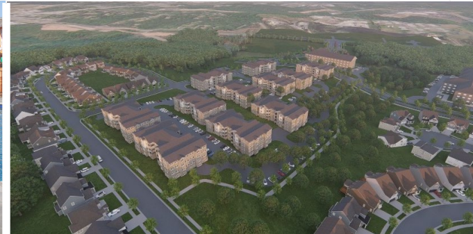
The Ridge at North Pointe (Great Eastern) 224 Units | Built 2023 Additional units underway
