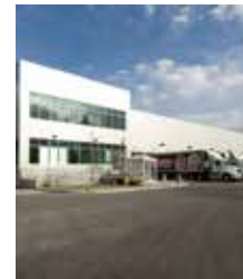
Dunkin' Northeast Distribution Center Bellingham, MA
