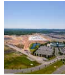
Logistics & Tech Park At Rentschler Field East Hartford, CT
