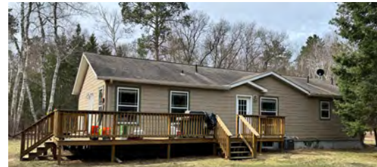
Ranger Residence and Office
