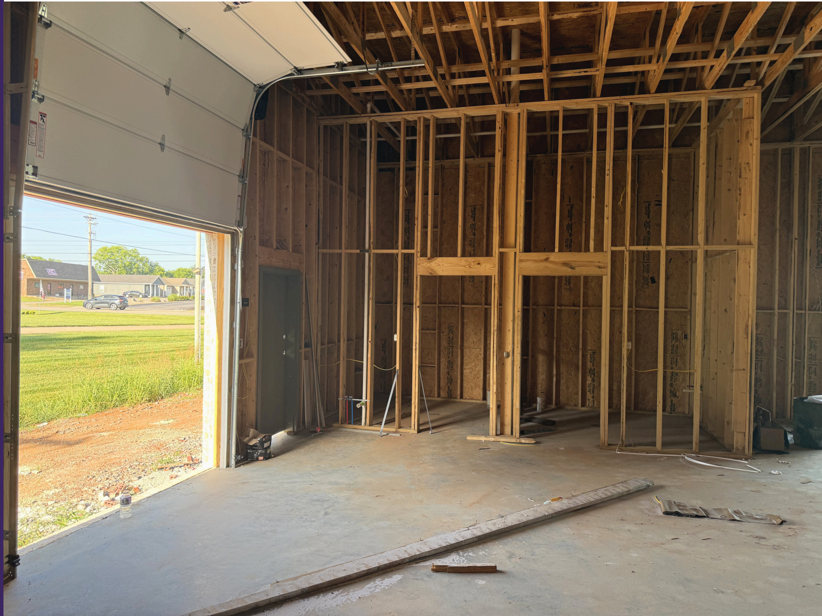
Main floor garage door
