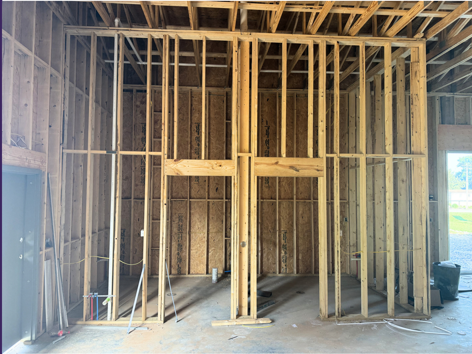
Main floor bathrooms
