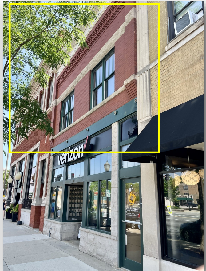
5 S. LaGrange Road, La Grange 2nd Floor Loft Office
