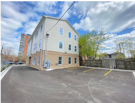
Rear elevation & private parking
