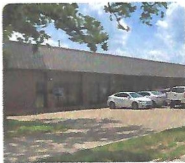
★ 2700 FINFEATHER Office / Warehouse
