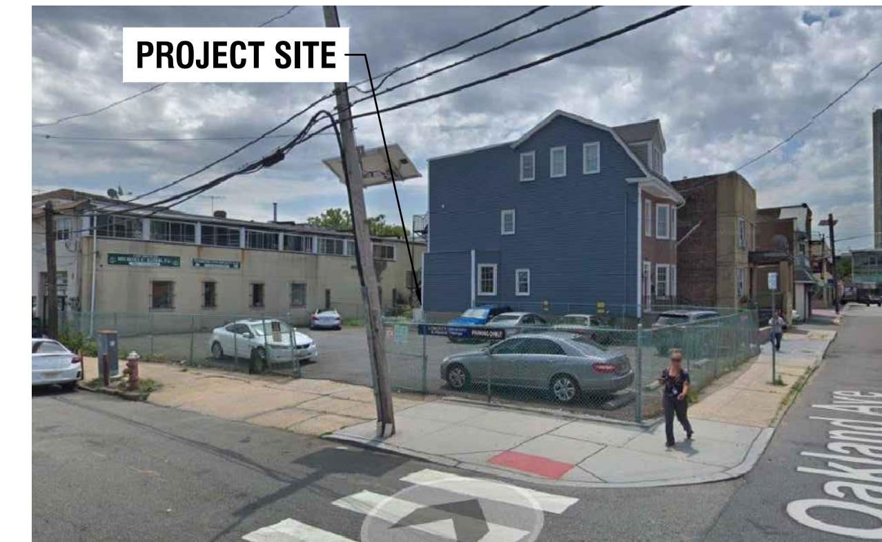
EXISTING SITE PHOTOGRAPH
