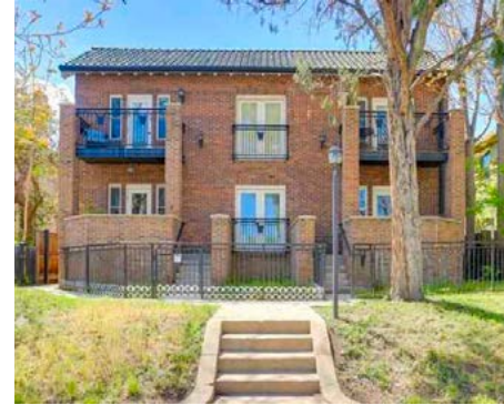
3615 FEDERAL BLVD Denver, CO 80211
