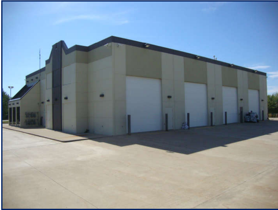
Rear View of Subject Property – Looking Southwest
