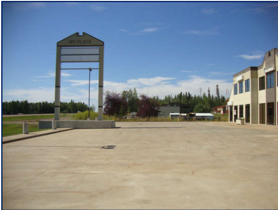
South Side Parking Area – Looking West
