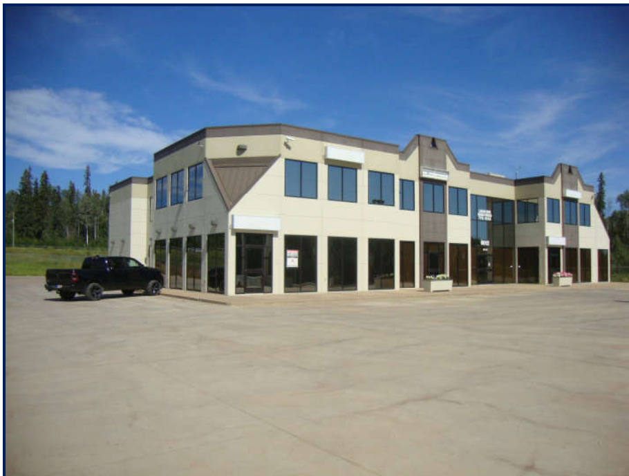
Front View of Subject Property – Looking Northeast
