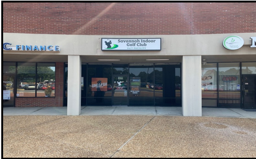
Northeasterly View (Front) Of The Southwesterly Elevation
