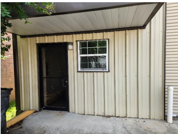
610A Office entrance
