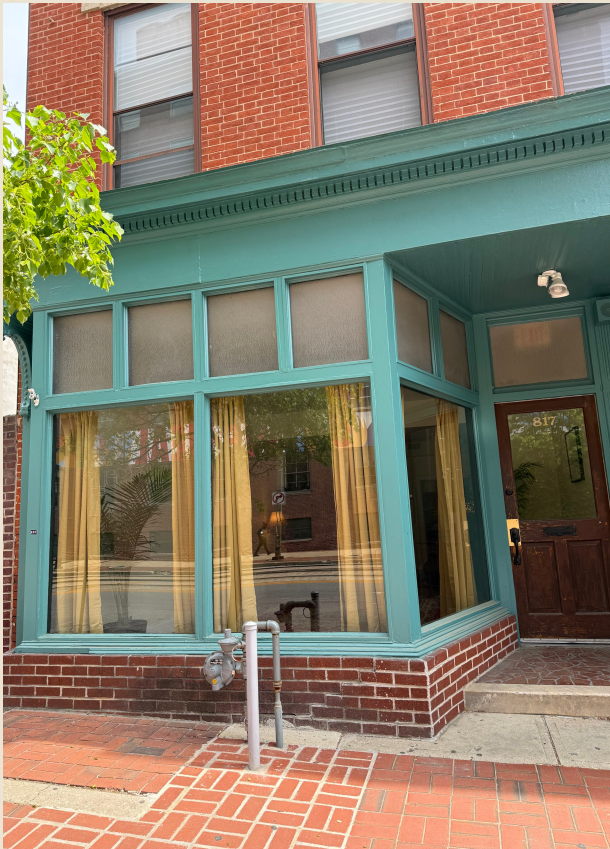
817 N Howard Street in daylight. Owner photograph.
