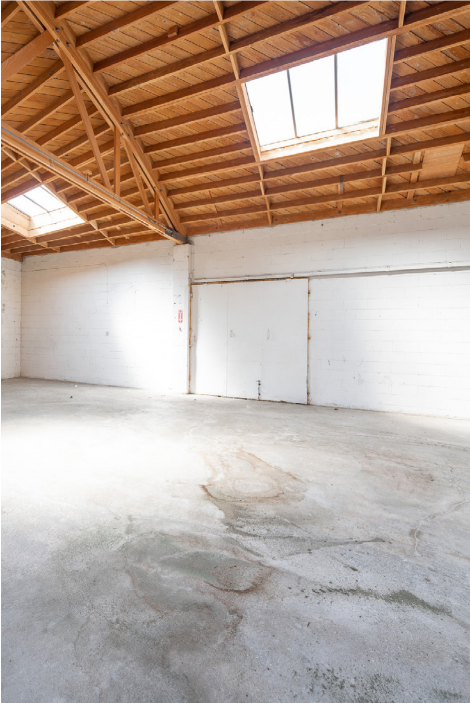
● Main warehouse floor
