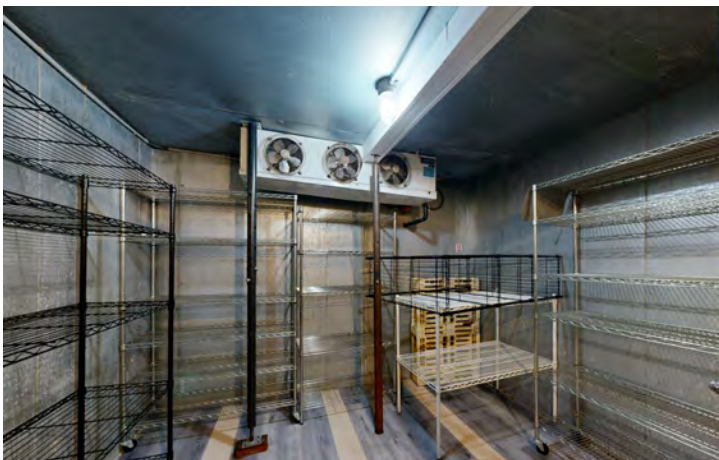
Walk-Out Lower Level For Storage With 11' x 14' Walk-In Cooler
