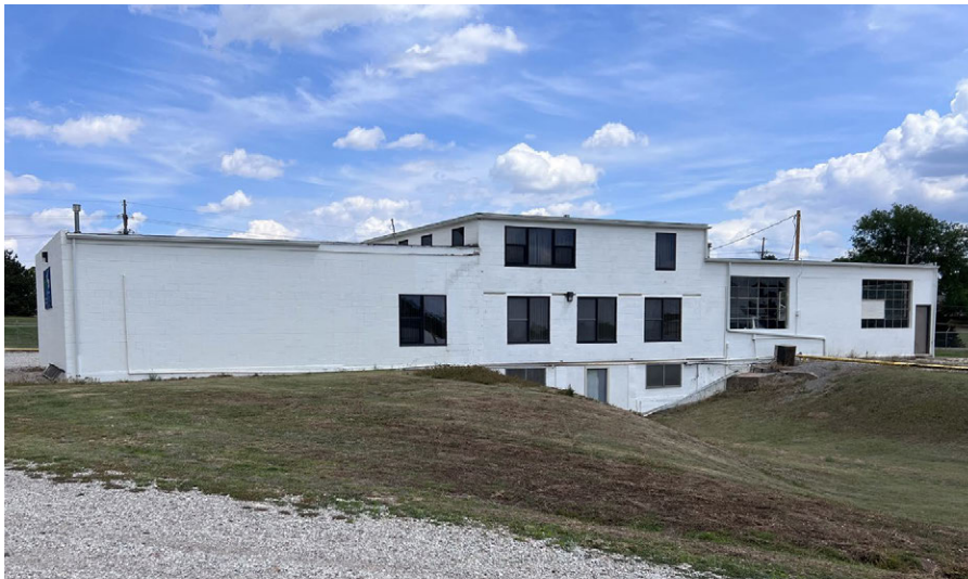
OFFICE WAREHOUSE REAR ELEVATION
