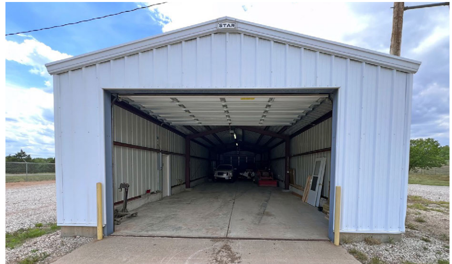
STAR PULL THROUGH BUILDING
