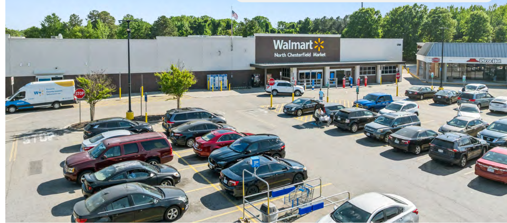
Recent Signage and Exterior Upgrade
