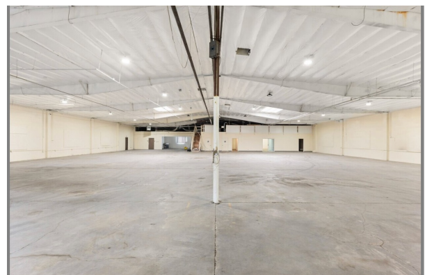
Warehouse interior — clear-span floor
