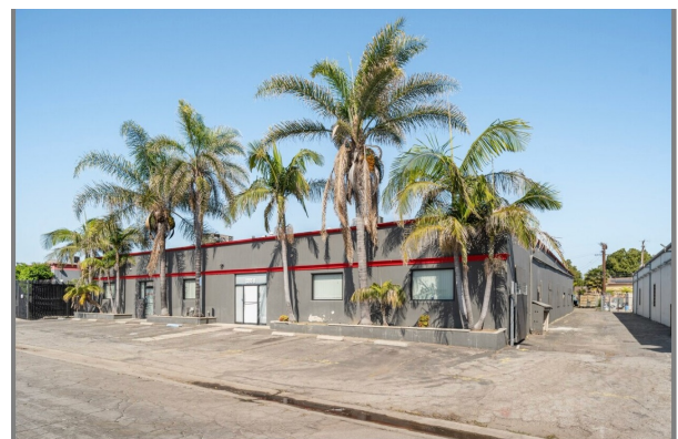
Building frontage — East 59th Street
