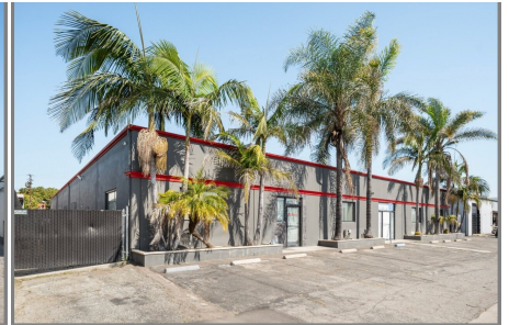
Exterior — west angle
