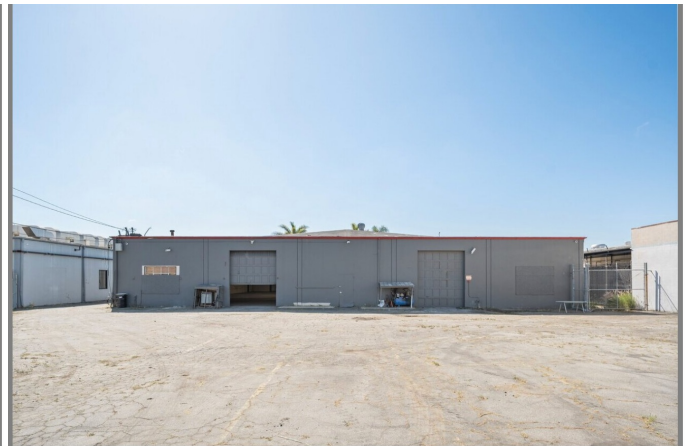
Rear yard — grade-level doors & secured yard
