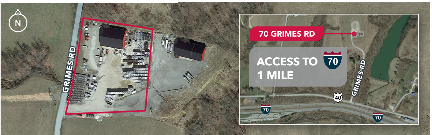
70 GRIMES ROAD - BUILDING A | CLAYSVILLE, PA 15323
