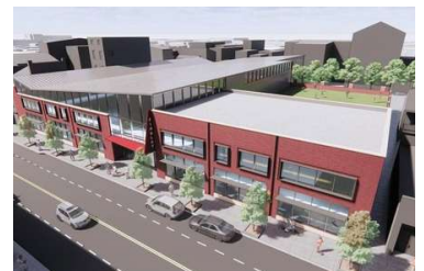
$61M OTR Project Findlay Community Center & Crossroads Health
